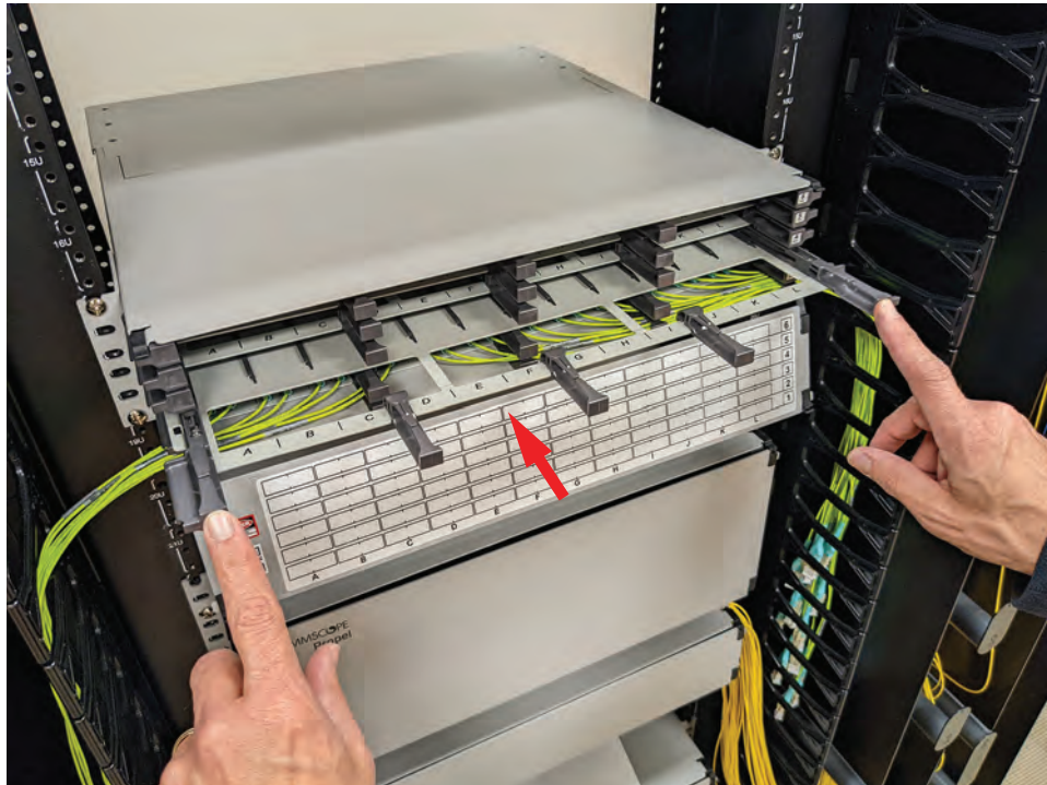
Figure 25. Installing a Blade
