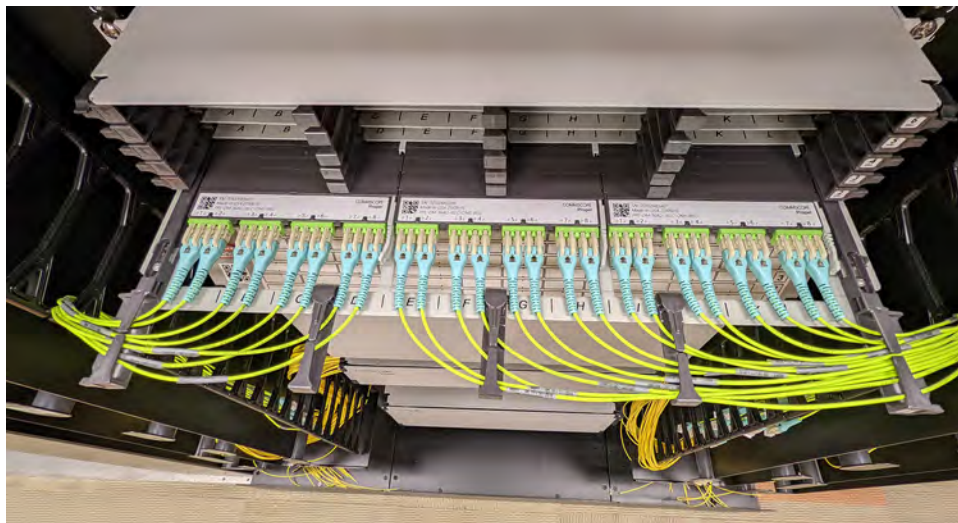
Figure 37. Patch Cords Fanned to Both Sides and Secured Within Patch Cord Managers
