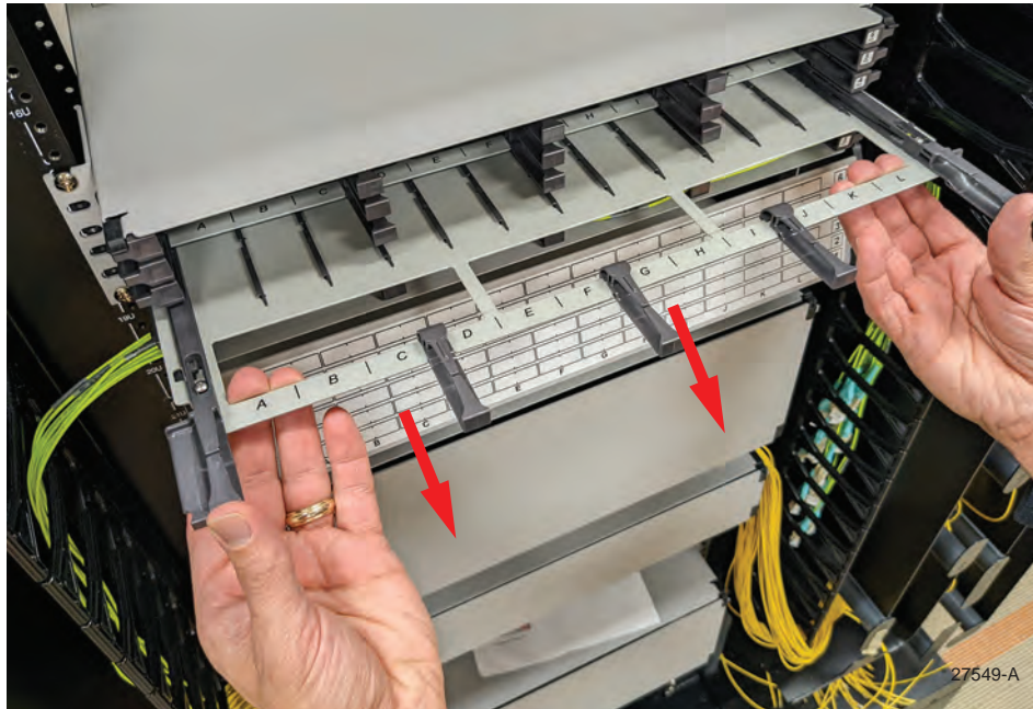
Figure 23. Hand Position to Release Blade
