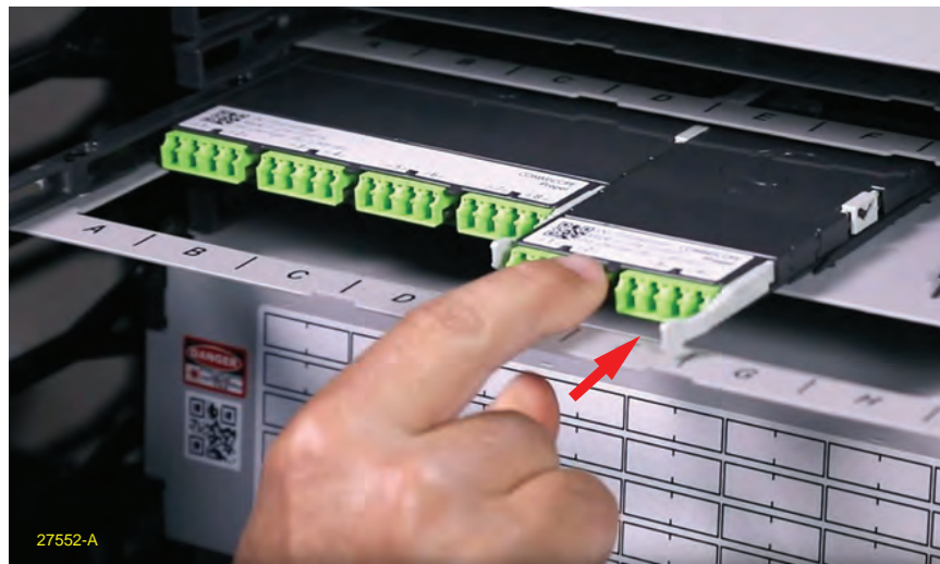
Figure 28. Installing a Connection Component
