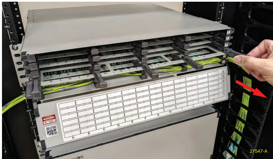
Figure 22. Sliding Out a Blade
