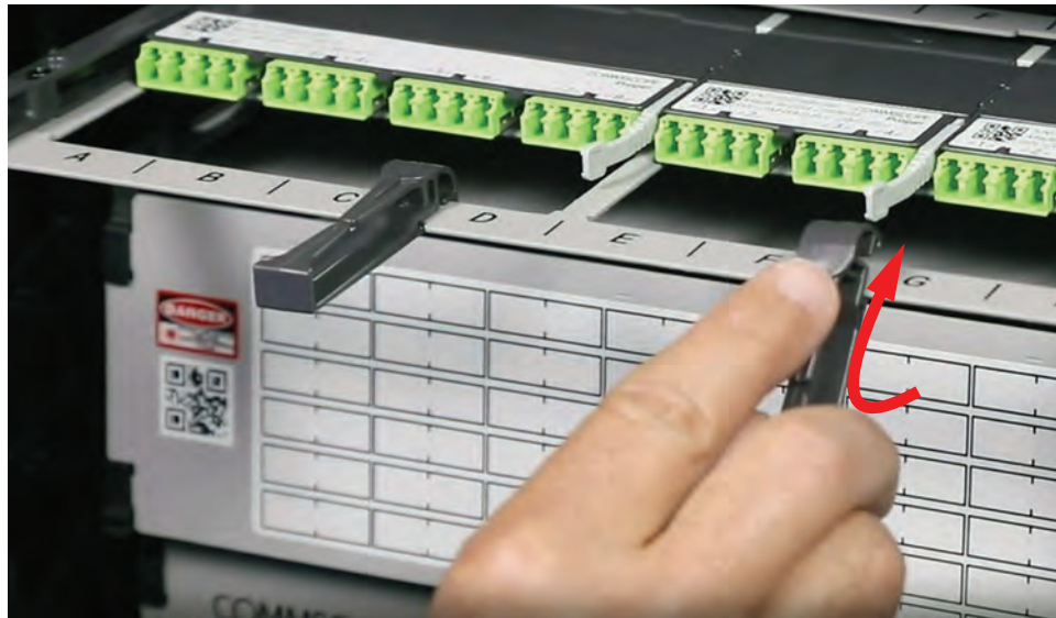
Figure 35. Inserting Patch Cord Manager in Notch
