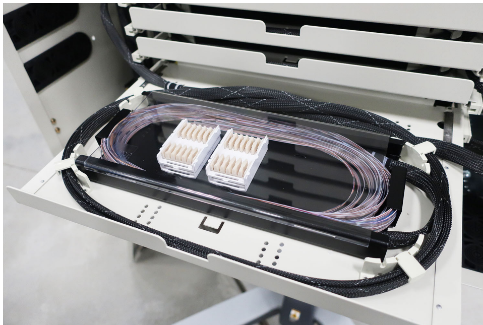
Figure 19. FST-XD-MT Splice Tray With 288 Fibers
