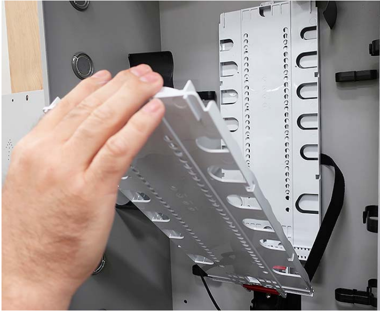
Figure 13. Installing the Second Splice Tray
