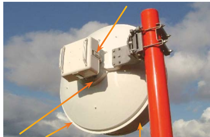
9.17: Example of RF leakage in a noncompliant microwave antenna
