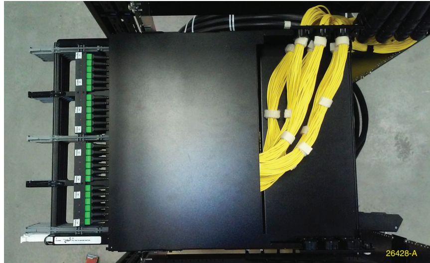
Figure 20. Single Entry Cable Routing (Top View)
