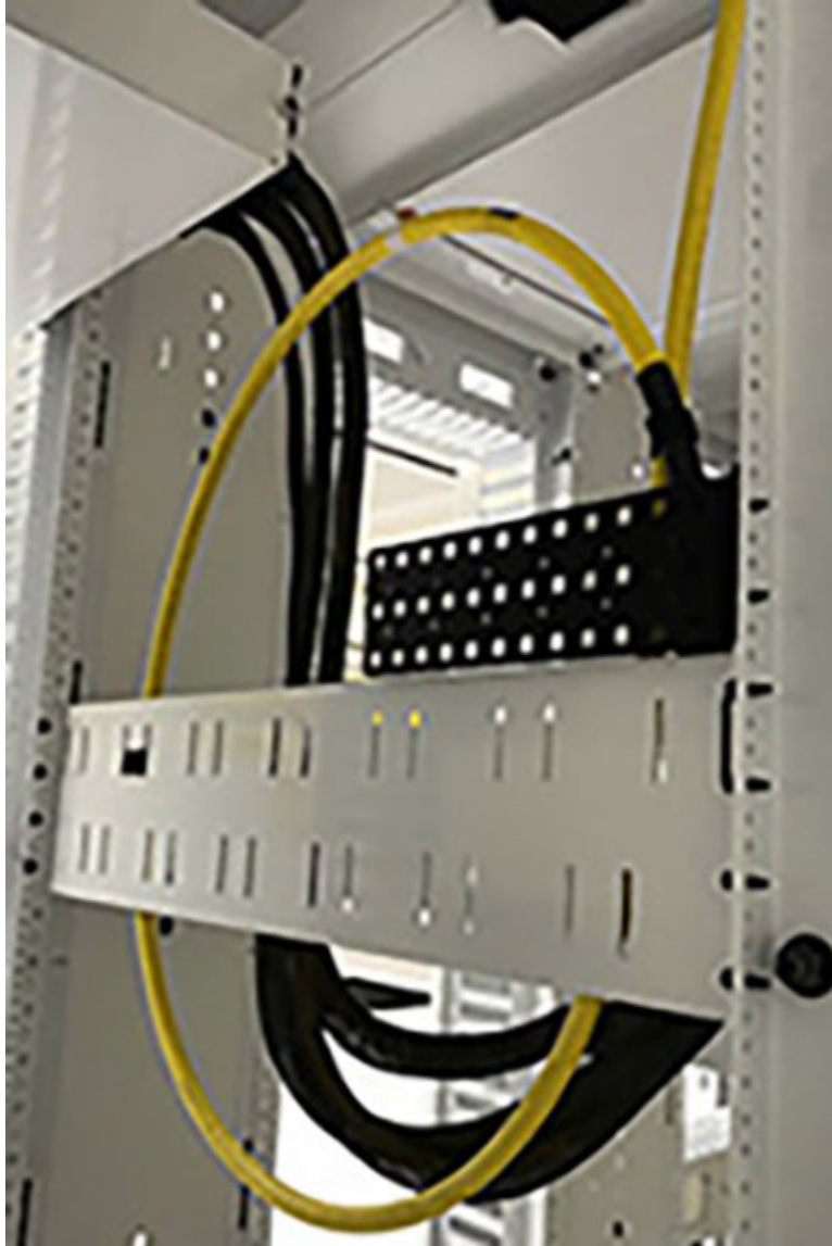
Figure 31. Drip Loop
