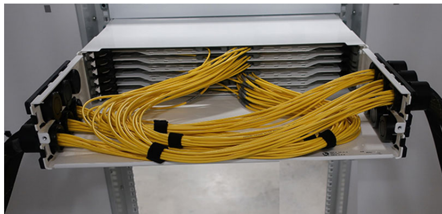
Figure 21. Left and Right Cable Routing (Rear View) (Cables With Hook-and-Loops Shown)
