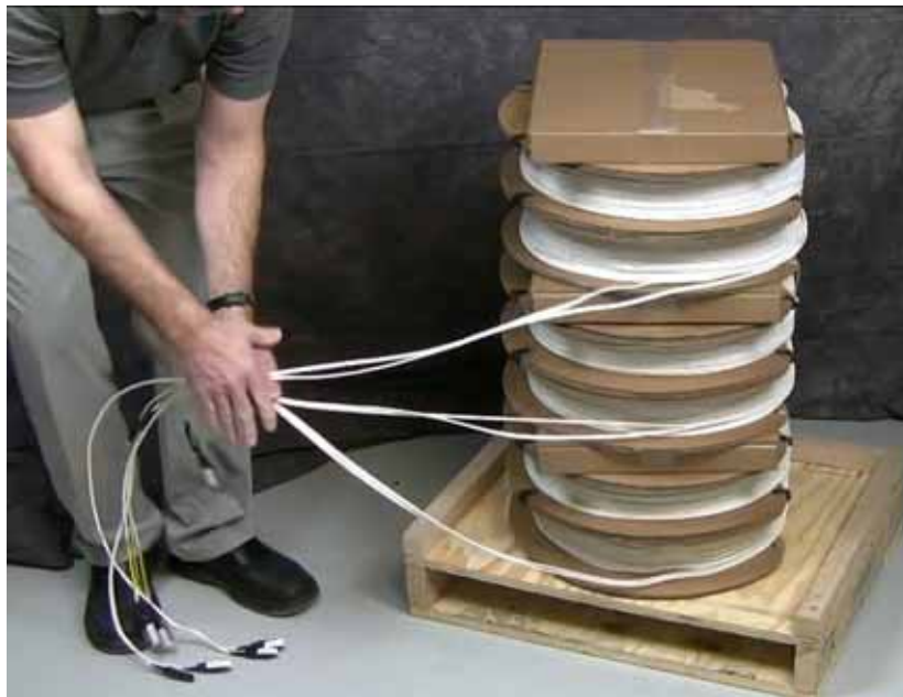
Figure 35. Proper Pulling Technique
