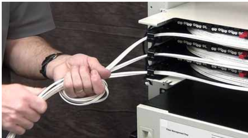
Figure 52. Hand-Wrap Method for Pulling Cable
