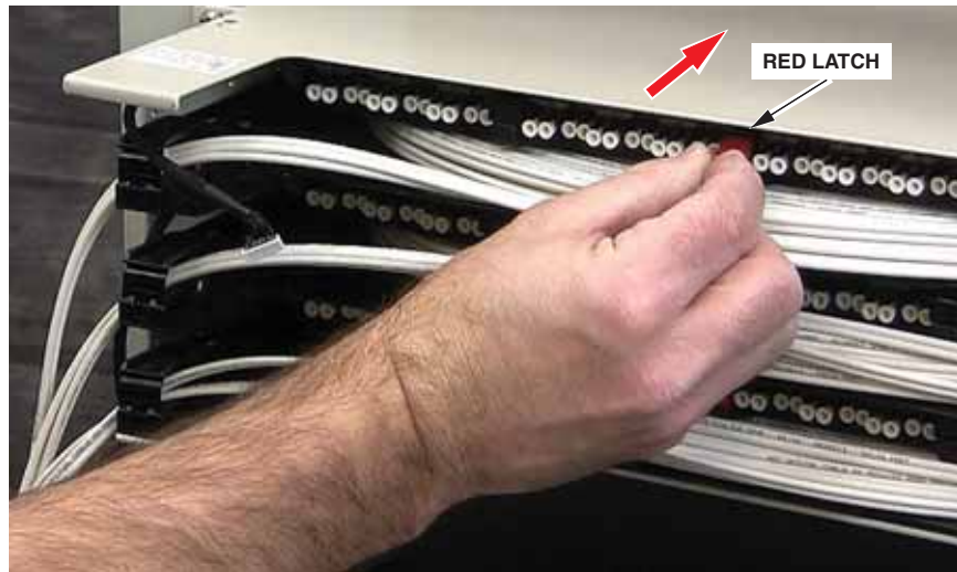
Figure 20. Locking Tray Into Pay Out Position
