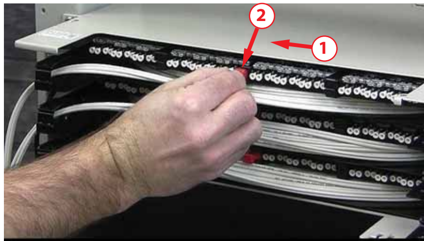
Figure 27. Pulling Tray Forward to Locked Operation Position
