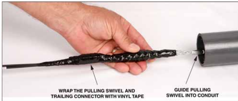
Figure 60. Wrap Pulling Swivel and Connectors with Vinyl Tape
