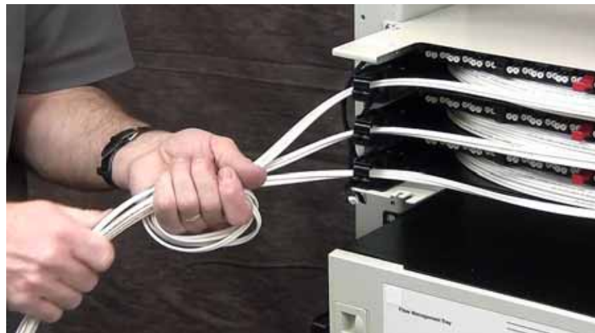
Figure 22. Hand-Wrap Method for Pulling Directly On Cable
