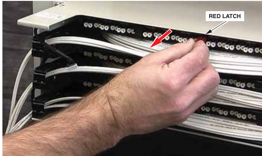
Figure 19. Pulling Red Latch Out to Release Tray
