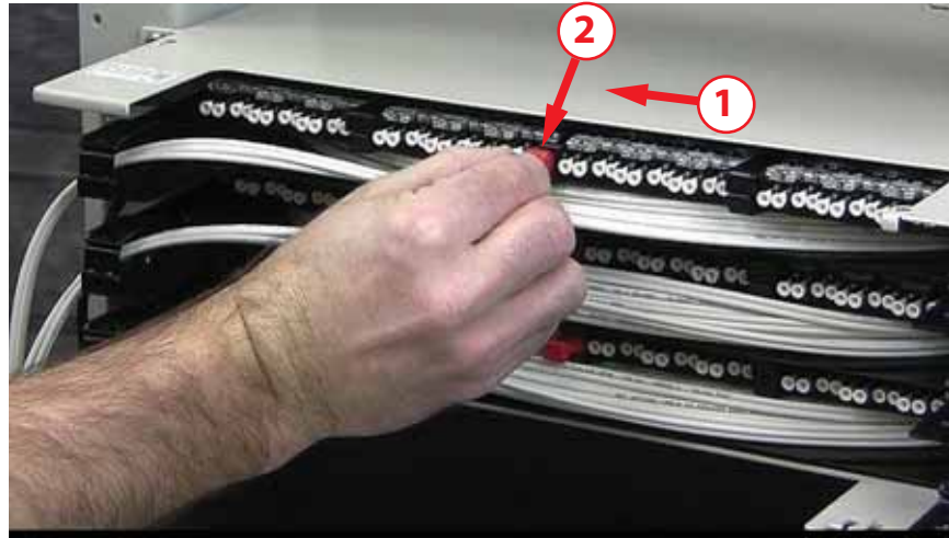
Figure 53. Pulling Tray Forward to Locked Operational Position
