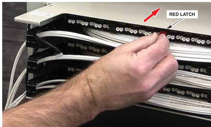
Figure 50. Locking Tray Into Pay Out Position
