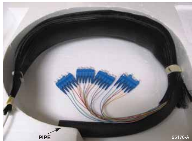
Figure 58. Remove Pipes from 900 mm Fanout Assemblies
