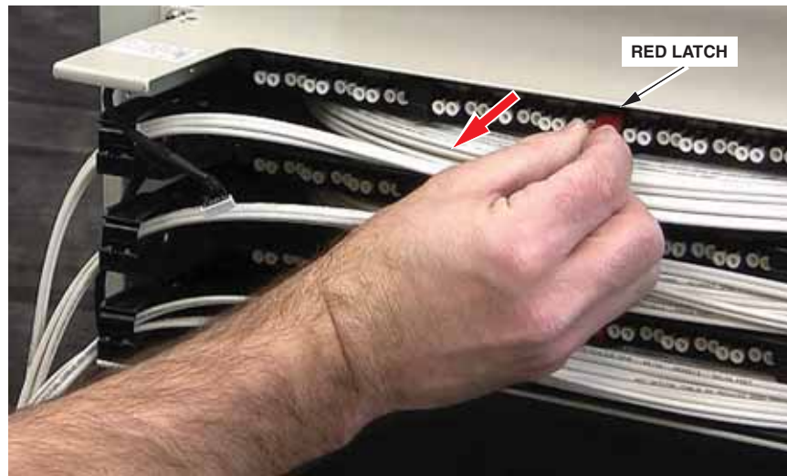
Figure 49. Pulling Red Latch Out to Release Tray
